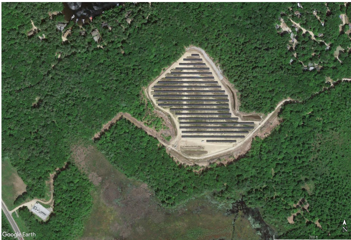
Figure 6: 2 MW NHEC Solar Project in Moultonborough, NH.
