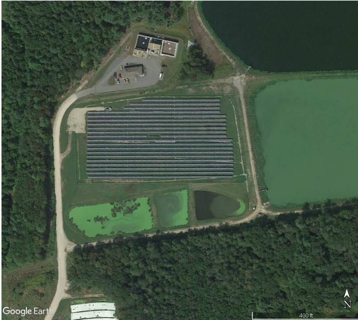
Figure 7: 0.9 MW Solar Project in Peterborough, NH.
